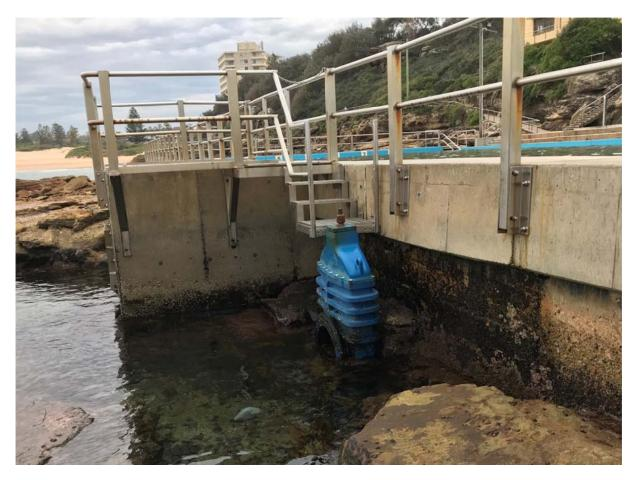
Figure 5.6 Gate valve for draining pool
