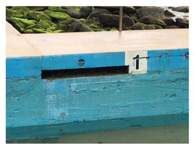
Figure 5.1 Stainless steel lane rope attachment and scupper
